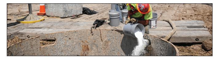
On smaller projects or mobile projects, such as Transmission Line and Cell Towers, BIG-FOOT may be added at the excavation by sprinkling carefully into a stream of water directed into the excavation or an agitator mix tank.
