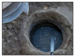
BIG-FOOT® Polymer Slurry is a soil stabilizing polymer. It is an easy mixing, 100% active polymer packaged as a granular powder. As the star of the BIG-FOOT® polymer SLURRY SYSTEM it is formulated to make a viscous slurry fluid fortifying the most challenging soil conditions.
