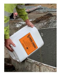
CRISS-CROSS® additive is a highly concentrated thinner that is effective with Bentonite drilling fluids. CRISS-CROSS works quickly to thin and disperse Bentonite fluids used in slurry diaphragm and cut-off walls. CRISS-CROSS is very effective at reducing the viscosity and gel strengths of freshwater drilling fluids.
