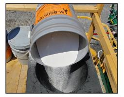
M-BOOSTER® Dry pH Adjuster is used to pre-treat the mix-water prior to adding BIG-FOOT® polymer slurry. It acts to insolubilize calcium from mix-water and groundwater. M-BOOSTER also functions to condition and soften mix-water and raise pH. M-BOOSTER regenerates BIG-FOOT polymer which has been damaged by extreme carbonate alkalinity.
